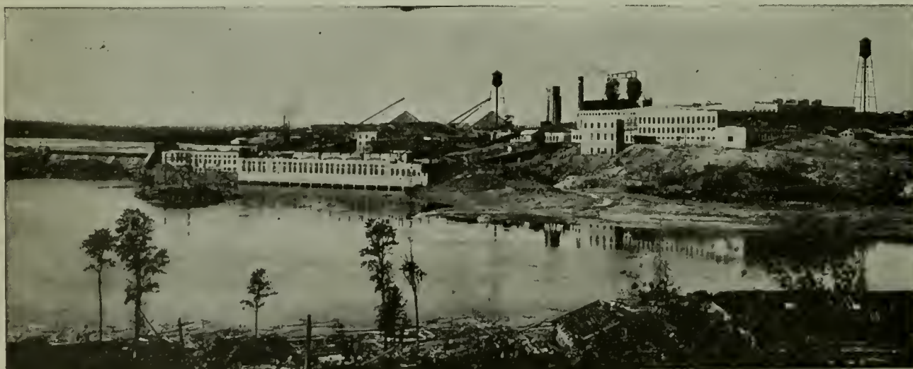
The mill of the Abitibi Power and Paper Company, Iroquois Falls, Ontario, showing from left to right the dam, the grinder and the mill. The capacity of this plant, probably the largest in the world, is 515 tons of newsprint and over 200 tons of pulp per day.
